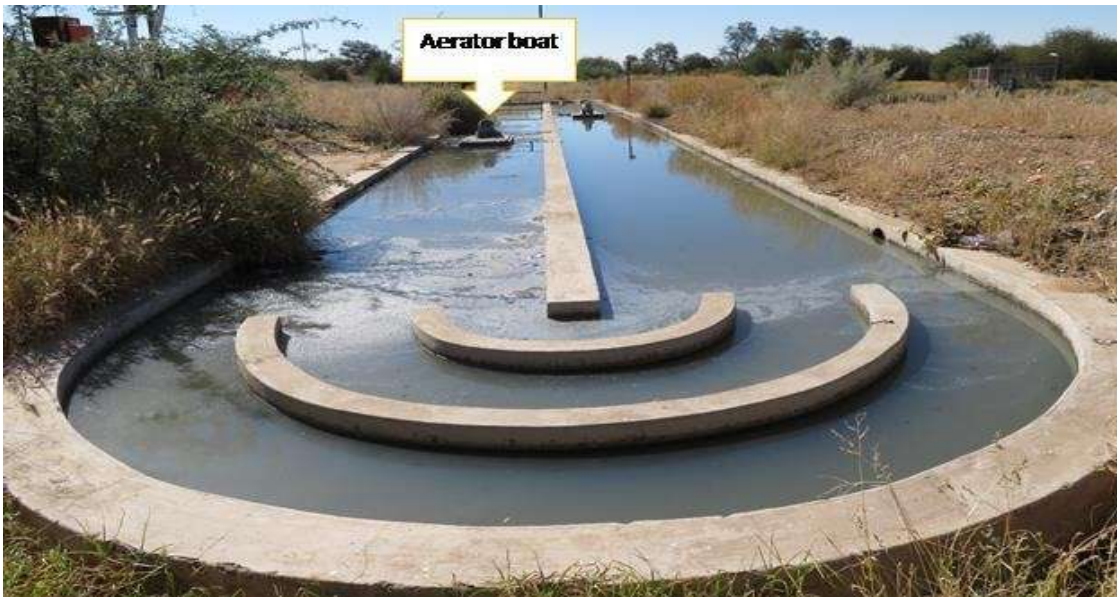
Figure 3. Sewerage settlement pond
