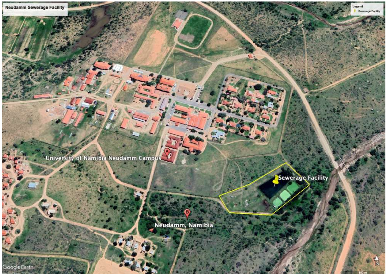
Figure 1. Neudamm Sewerage facility
