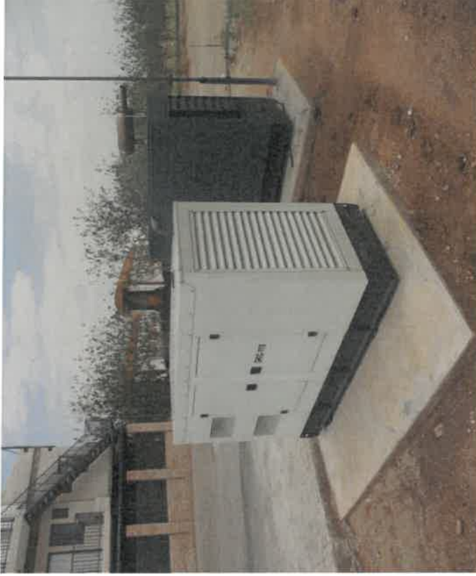
Figure 6; A diesel engine generator at the facility
