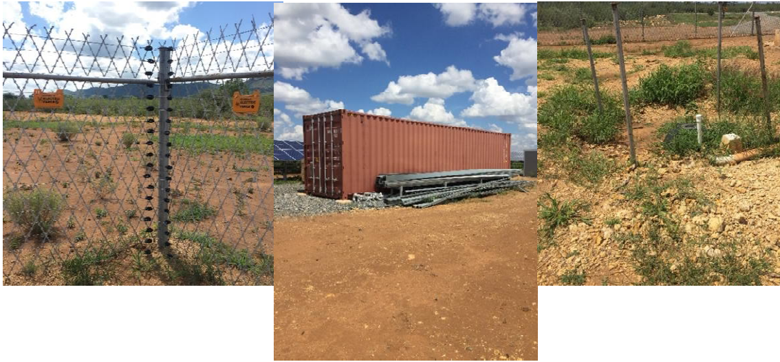
Photo set 2 Warning signs on fence, storage conditions, septic tank soil conditions.
