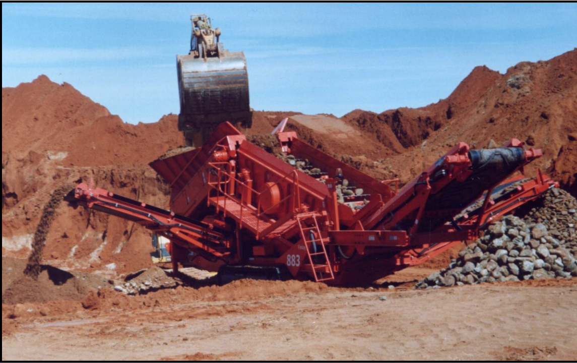
Figure 7: Example of an excavator feeding material into mobile screening plant and producing screened product stockpiles
