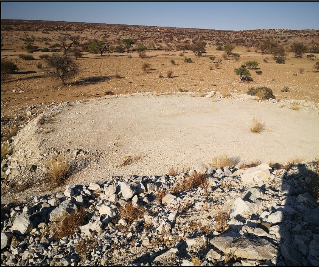
Figure 3: Stockpile of material blasted and excavated from the quarry
