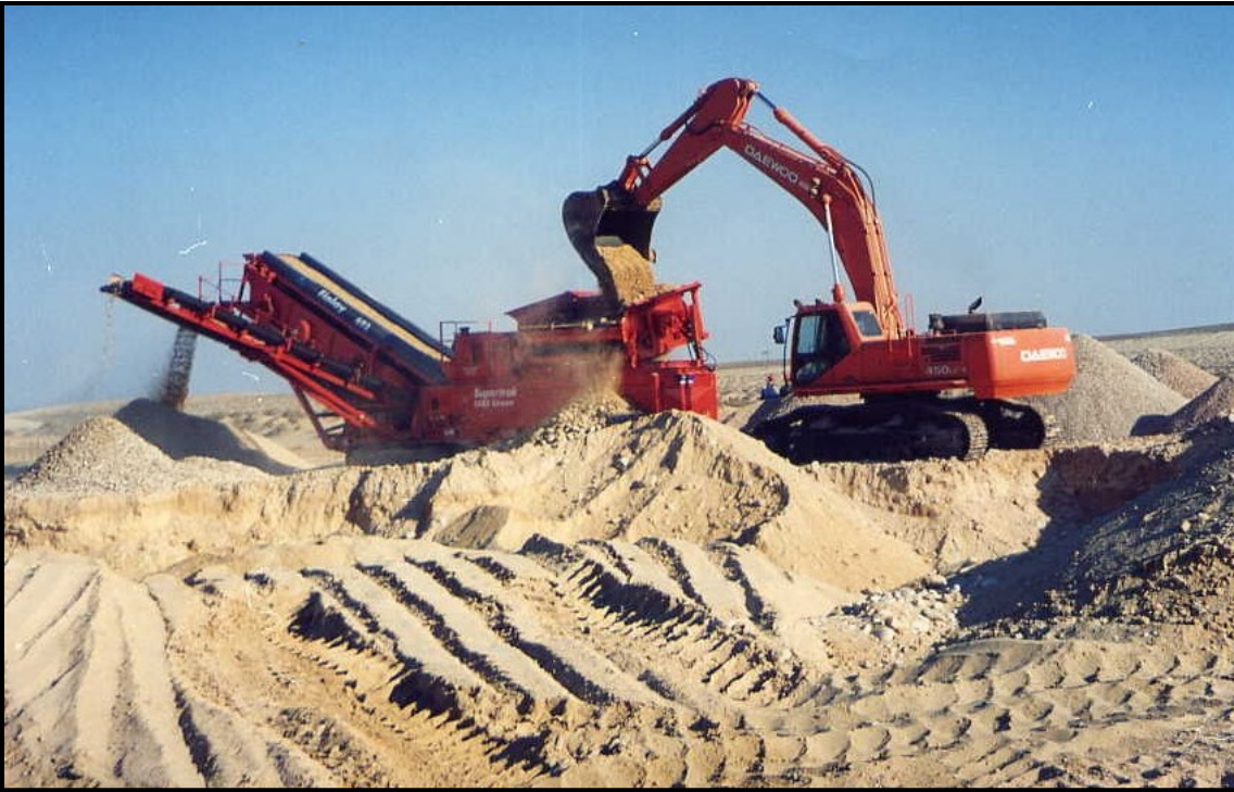
Figure 6: Example of excavator feeding material into a mobile screening plant
