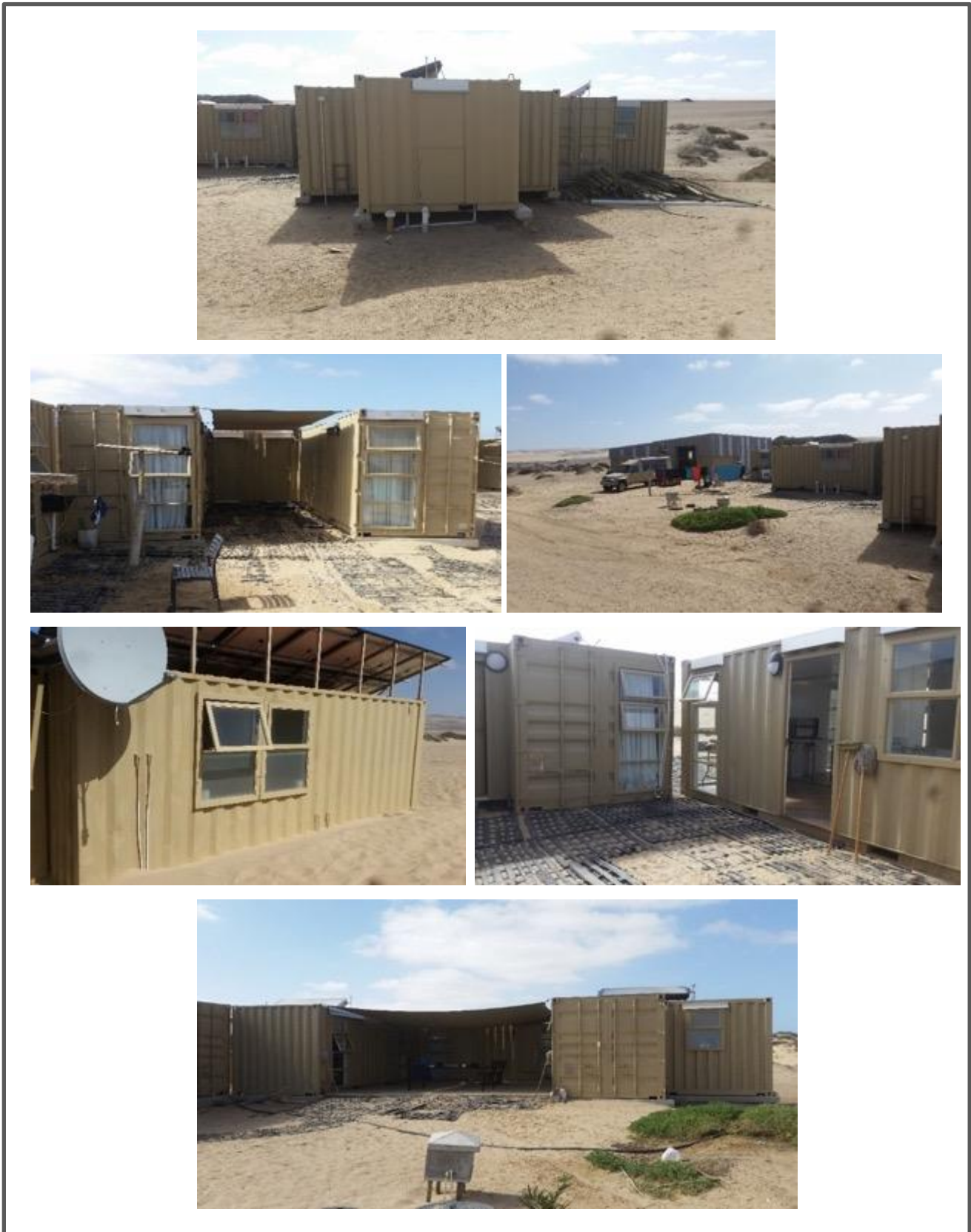
Figure 9. The staff village and workshop complex is built entirely from shipping containers.
