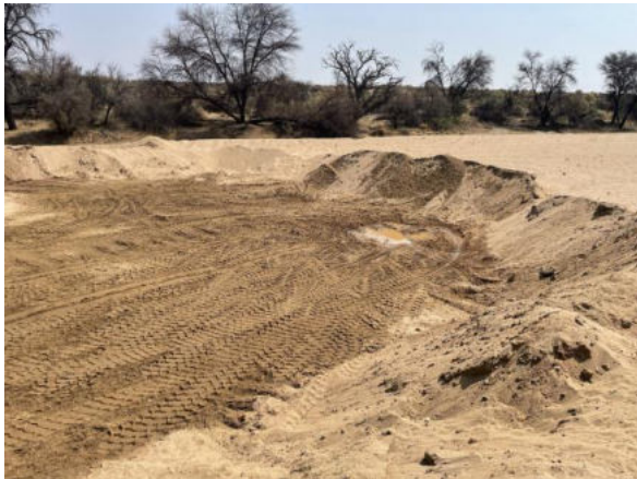
Photo 4-7 Sand buffer between Schaaf River and active mining operation
