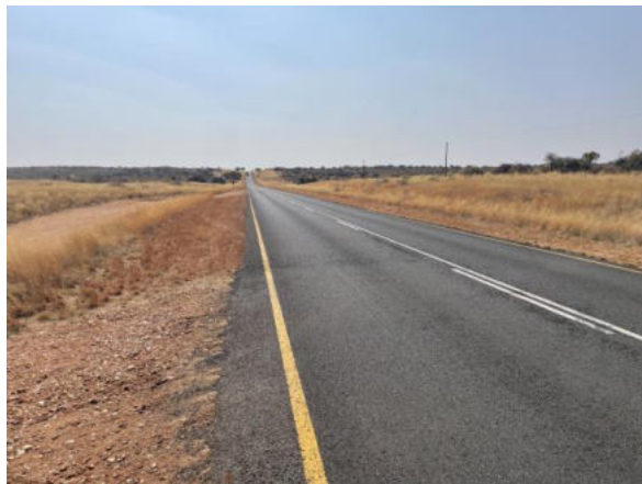
Photo 4-11 View from the entrance onto the C23 towards Windhoek
