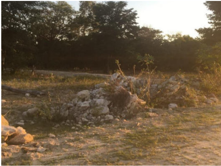
Figure 4: Gravel Road construction works in 2021
