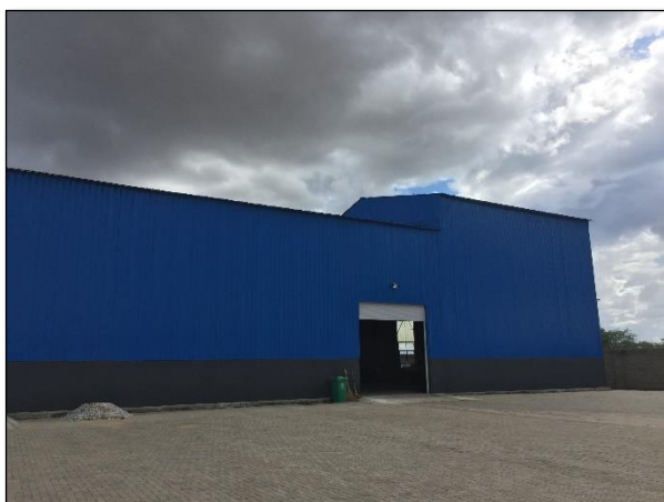
Figure 2: The Existing Waste Car Battery Recycling Factory
