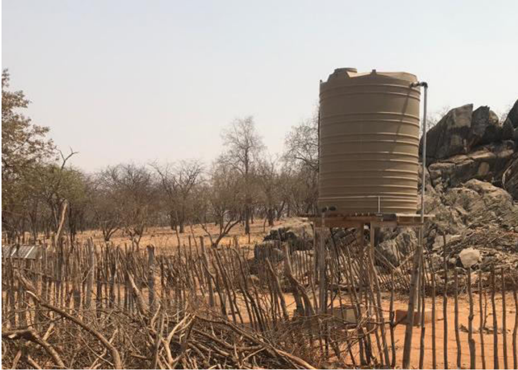
Figure 4: The borehole (water source) observed during site visit
