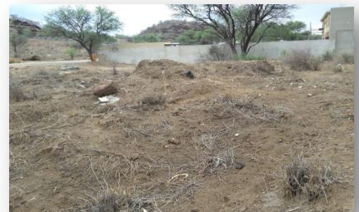
VIEW (2) OF THE SITE- BUILDING RUBBLE AND ERF WORKS
