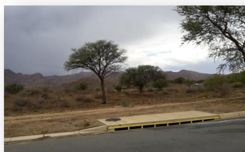
VIEW (4) OF THE SITE – HYDROLOGICAL INFRASTRUCTURE
