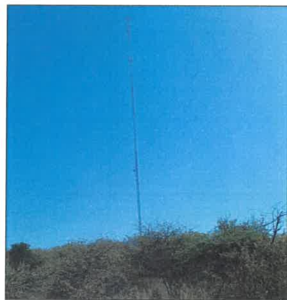
Image 1-4: Telecommunication tower in project area
