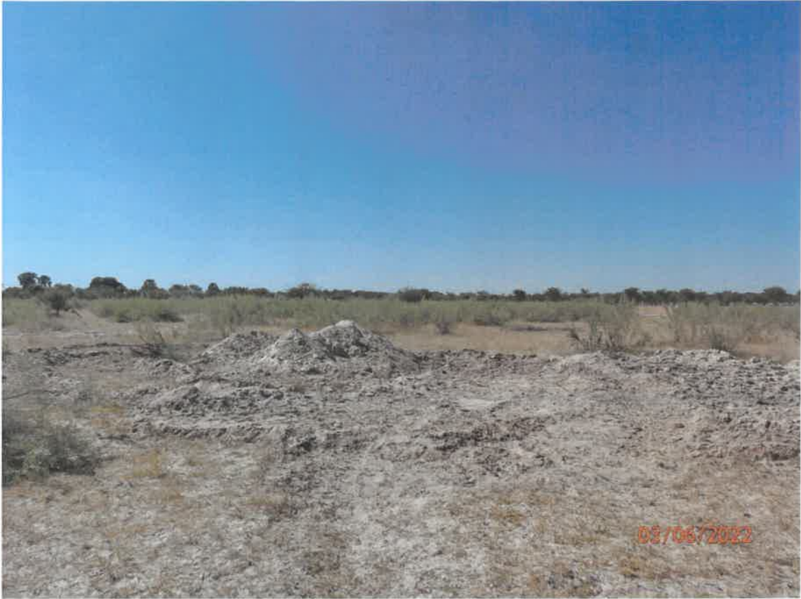
Trial pit for testing if the soil grade is suitable for road construction
