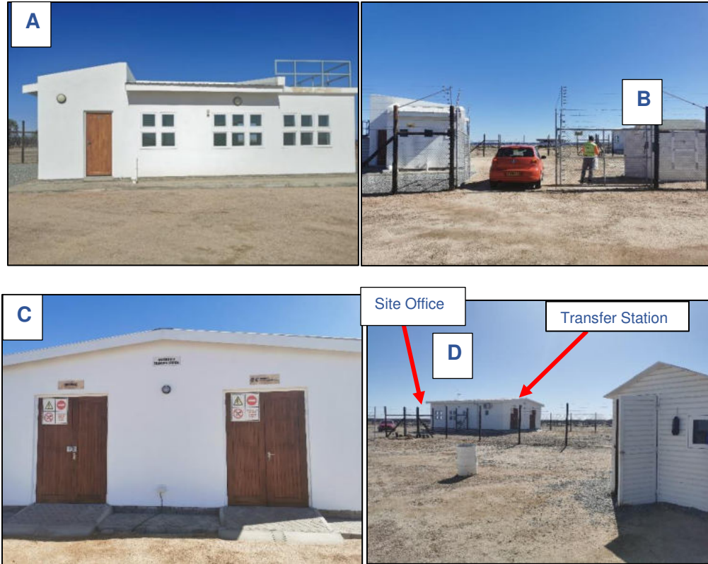
Figure 2-9: Site structures (A- Training Centre, B -Security Control, C- OLC Transfer Station (eastern side), D – Site Office (western side)
