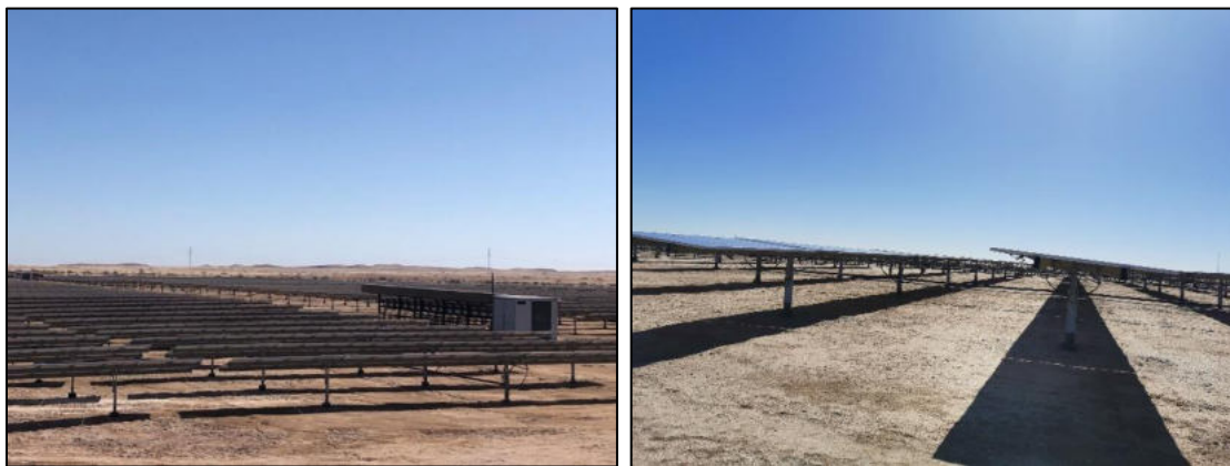
Figure 2-1: Some of the solar panels at the OLC Arandis Solar Energy Plant Site
