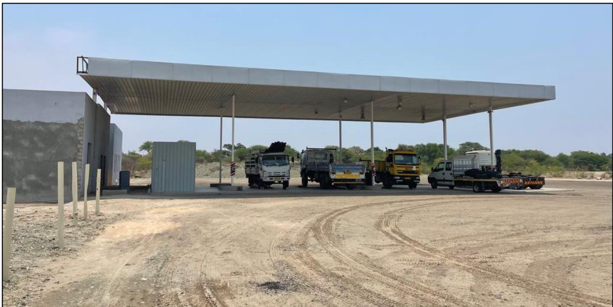
Figure 4: Photo of operations on site
