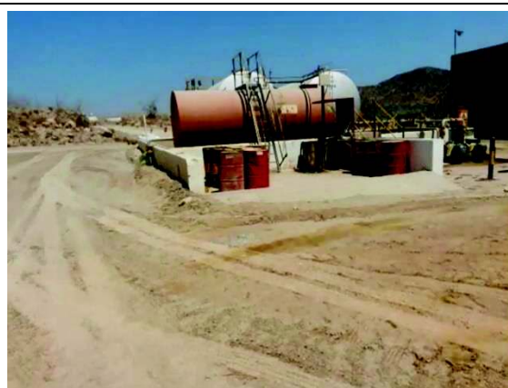
Photo 2 Used oil tank and diesel storage tanks.
