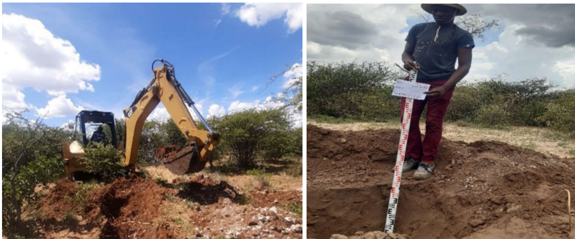
Figure 2.1: Borrow pit investigation
