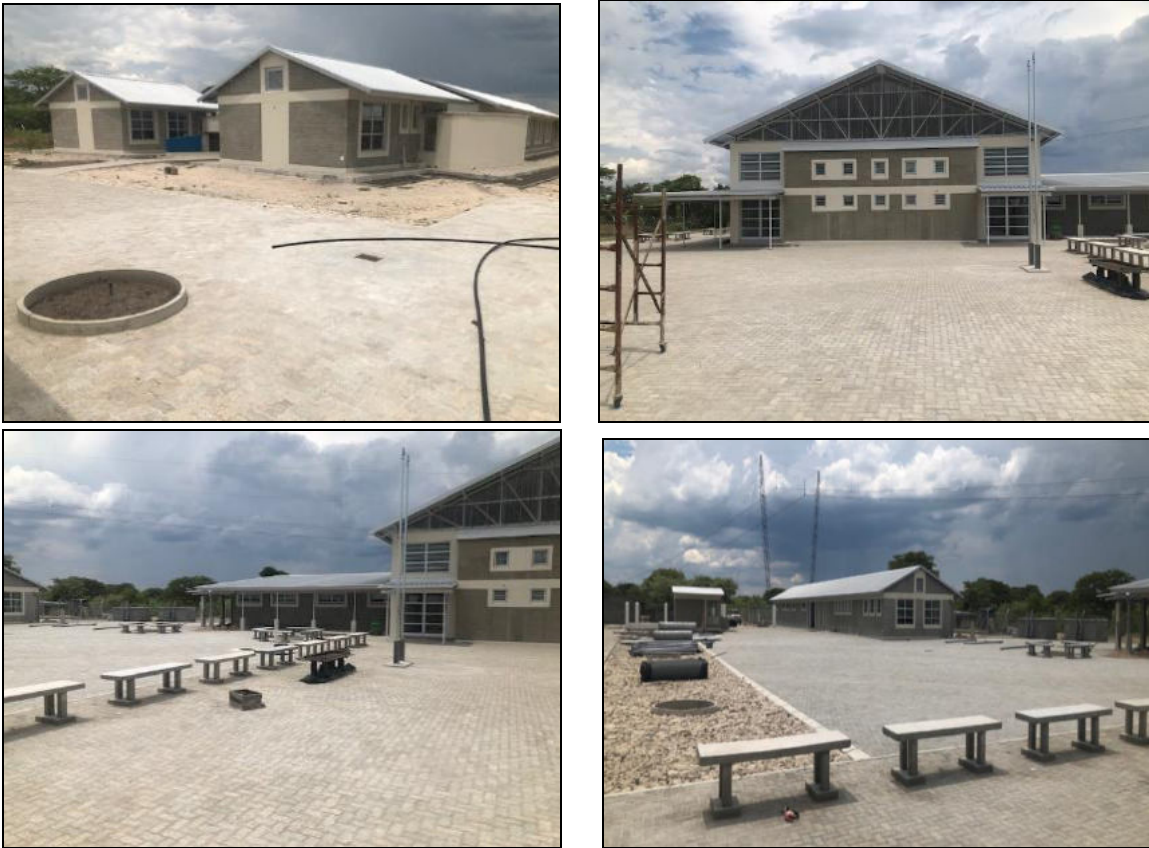
Figure 4: New hostel facilities already constructed at the School
