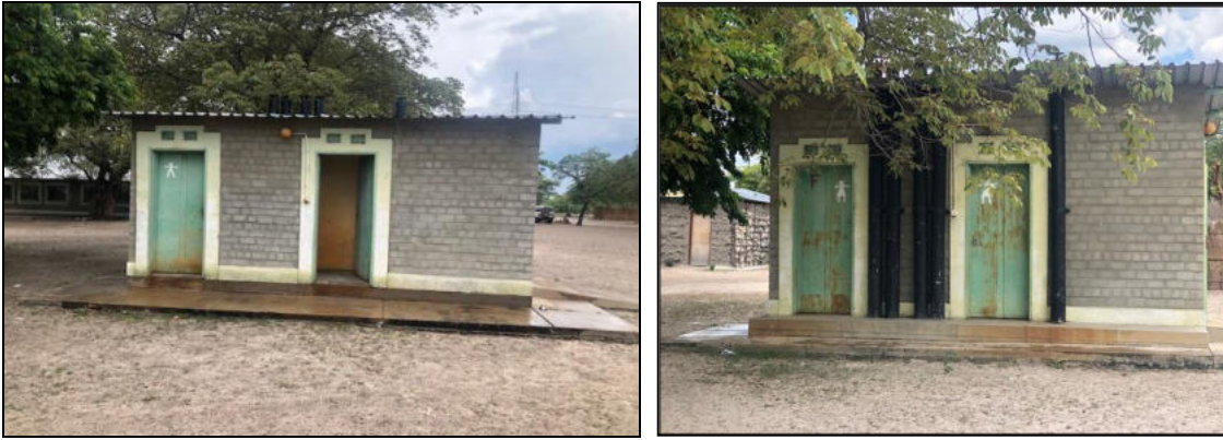
Figure 3: Existing facilities on site
