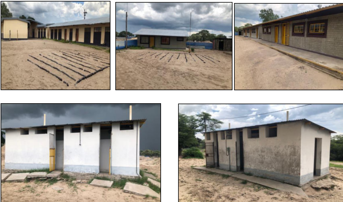
Figure 3: Facilities on site
