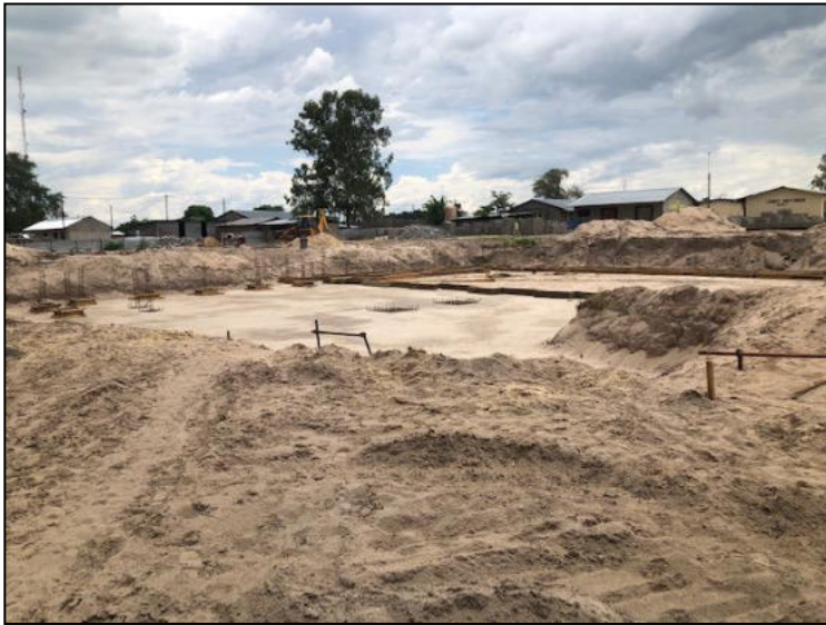
Figure 5: Photos showing the progress with construction
