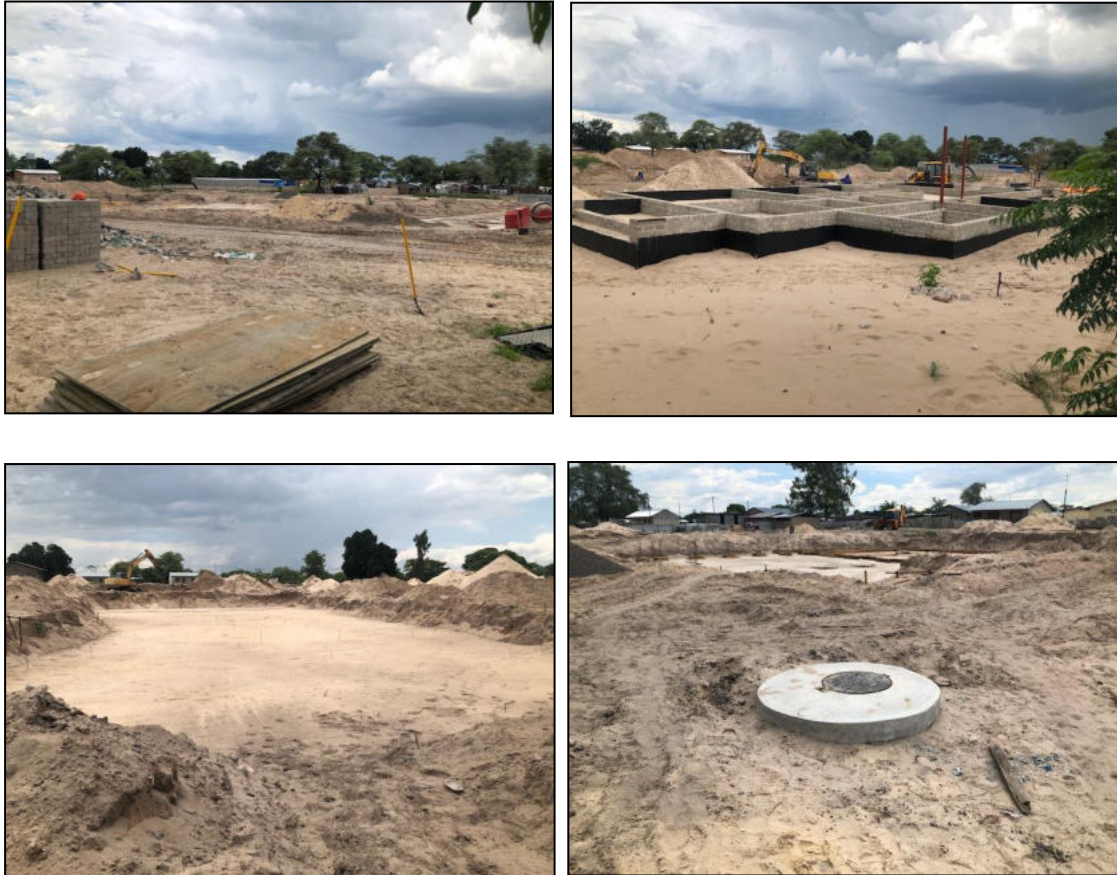
Figure 4: New infrastructure being built
