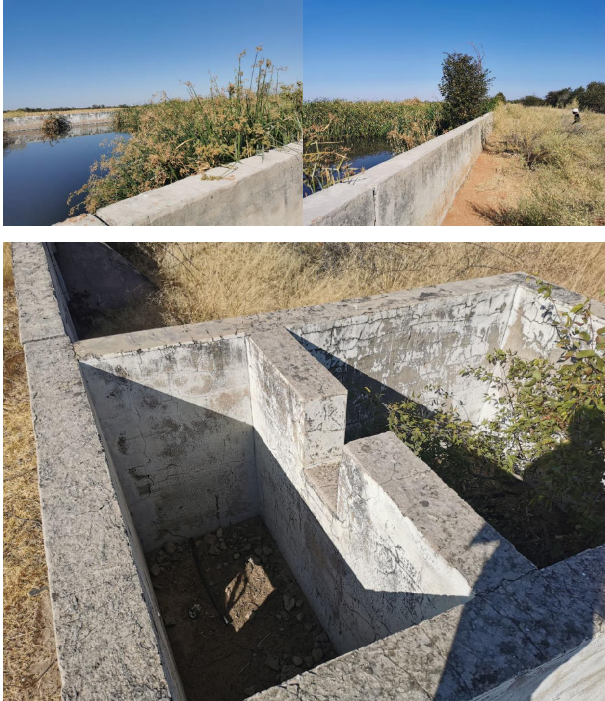
Figure 2-1: The current status of the oxidation ponds in Oshifo Town
